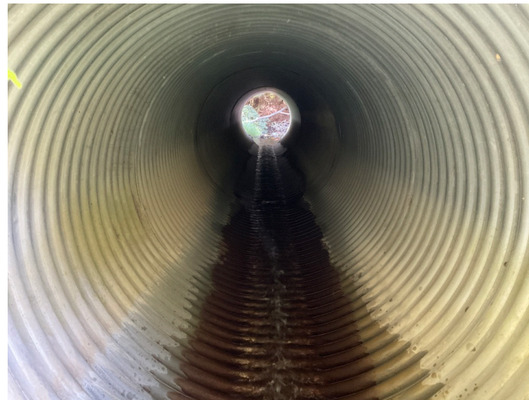
Looking Downstream Through CMP
