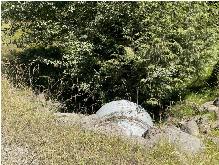
Upstream from Crossing
